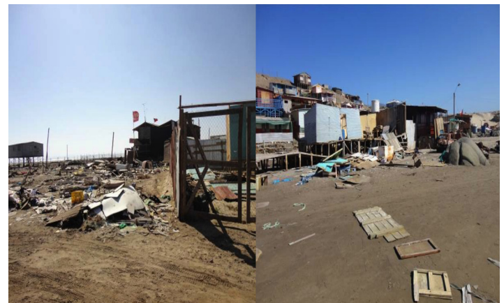
Fig. 2. Images of destruction in Puerto Viejo by Japan's tsunami of March 2011.
