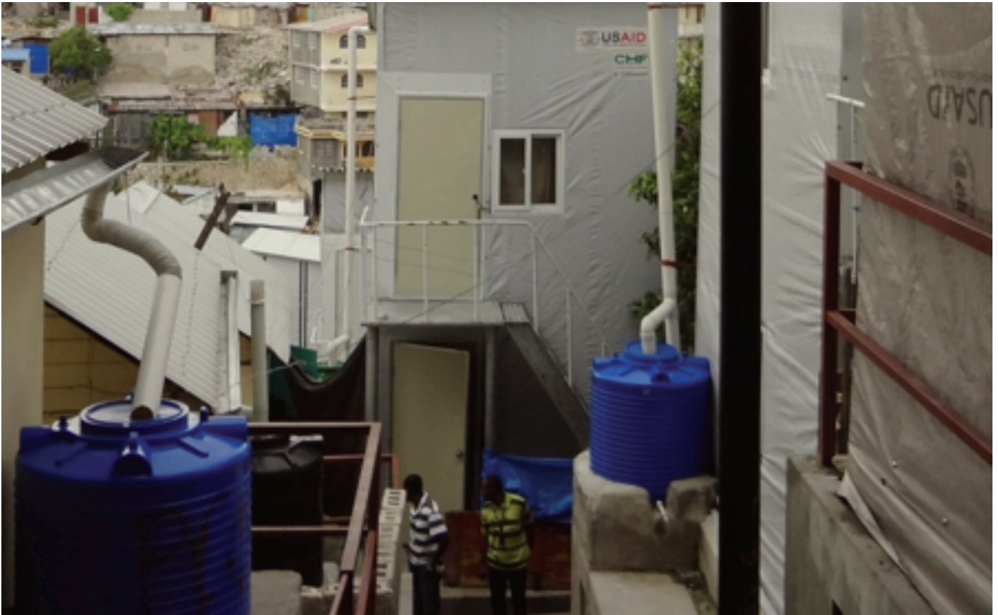
"PCI Neighborhood Approach Project in Ravine Pintade (Haiti): transitional shelters, access road, retaining walls, rainwater collection, solar street lighting, and drainage systems." Photo: J.P. Sarmiento
